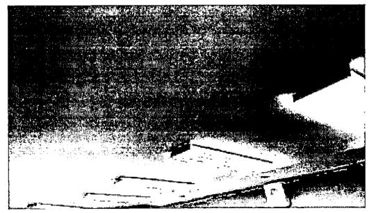
Removed old sealant, cleaned, and prepared glass panels and frames for new sealant. Resealed and replaced all silicone bridge sealant to fully repair leaking skylights at Liberty Elementary.
