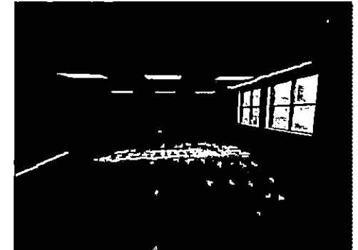
Removed Broken VCT & Installed 2x2 Grid System in Wrestling Room
