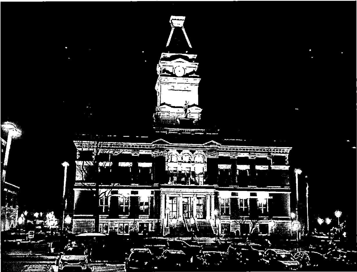
Historic Courthouse – New Lighting
